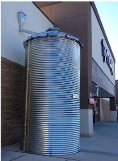
A 5,300 gallon tank for catching rainwater Corpus Christi, TX
