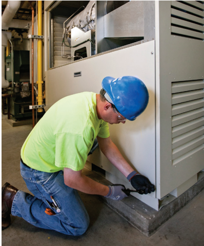
Installing the Capstone C65 microturbines
