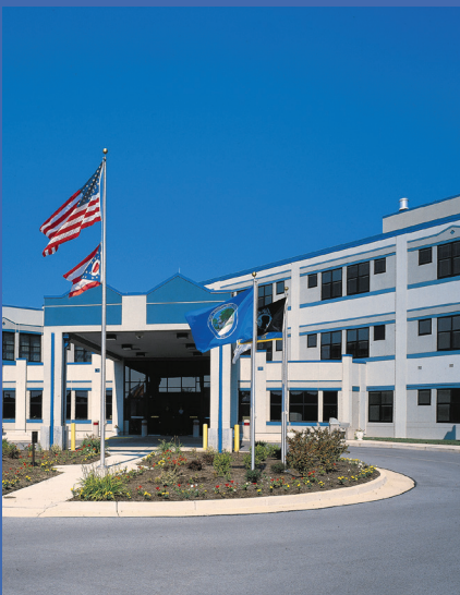
Highland District Hospital, a 25 bed critical access hospital, located in Hillsboro, Ohio
