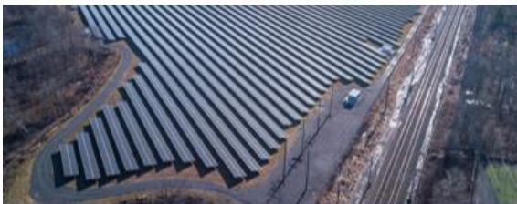
Old Bridge - 10.7 MW
