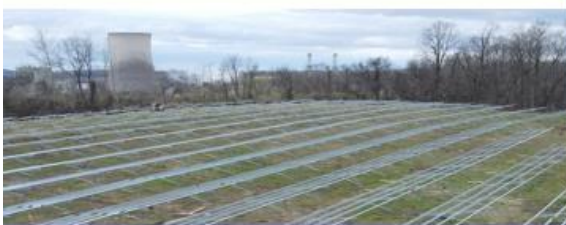
Foul Rift - 19 MW Under Construction
