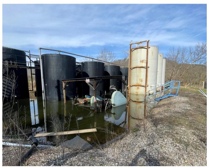
The Frost Well is on State Route 144 only 500 feet from the Hocking River in Athens County, Rome Township. The injection well leaked into production wells. Eventually it was suspended and the owner walked away leaving this mess.
