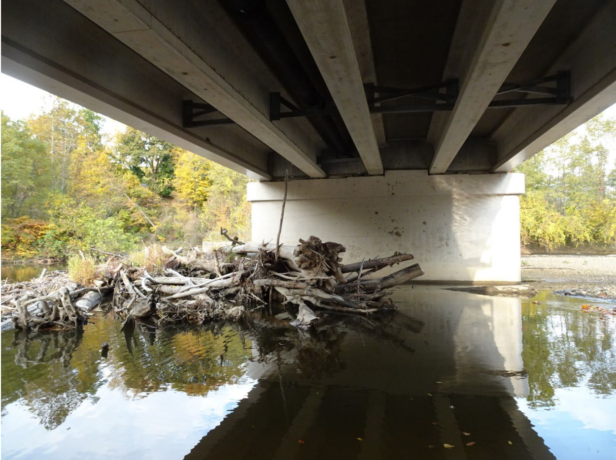
Bridge Carrying SR 84 Over Grand River in Lake County, Ohio:
