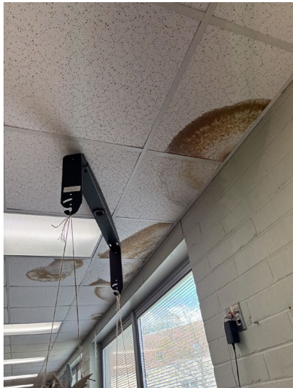
Water damage from roof at Windham Branch. This location, housed in a former school, has seen repeated temporary closures due to a faulty HVAC system.
