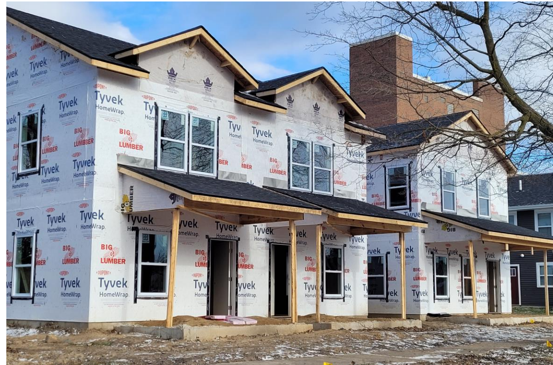
Pre-approved duplex under construction in South Bend, IN.
