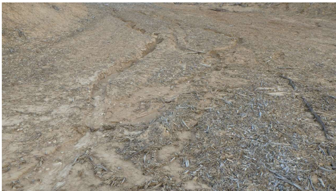
PHOTO 2 – Erosion gullies developed in short access road to a field. These erosion gullies have a cumulative length of about 600 feet and flow into a small road ditch with intermittent flow. Ohio EPA's new General Permit requirements effective June 2020 would apply to mitigate the filling of these ephemeral streams at an exorbitant cost (as much as $650 per foot).
