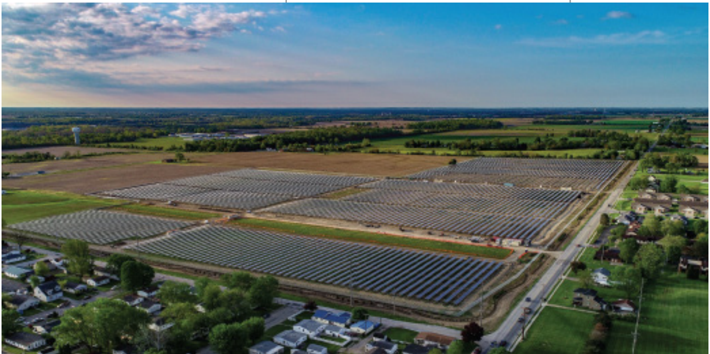
Piqua Manier Solar in Miami County
