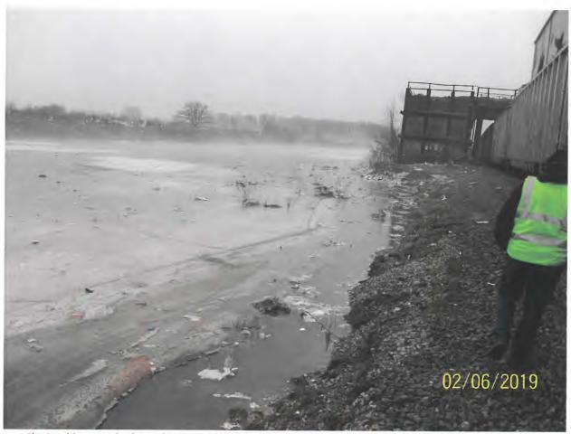
4) Looking south along the western edge of the east pond. The outlet end of the drain pipe is in the distance amidst the excessive litter and debris that has collected in the pond.
