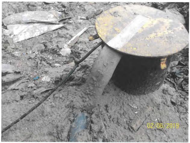
Capped riser pipe located at the northeast corner of the rail unloading building. Power cord, flexible hose, and edge of the hard pipe that continues under the tracks are displayed.
