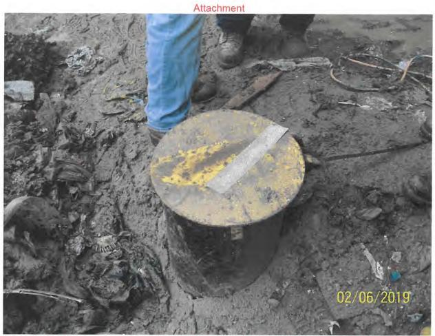
1) Capped riser pipe located at the northeast corner of the rail unloading building which housed the pump and flexible discharge house.
