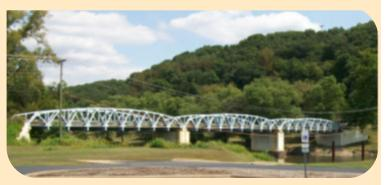
continuing accident problem. The existing bridge is only 24 ft. wide between trusses, and there have been numerous minor side-swipe accidents on the bridge as well as several accidents on the adjoining roadway. The realignment is done to address the deteriorating bridge condition as well as the adjacent roadway. In addition, the project will include sidewalk access for numerous pedestrians that currently use the 24 ft. wide bridge to access commercial establishments and trails.
